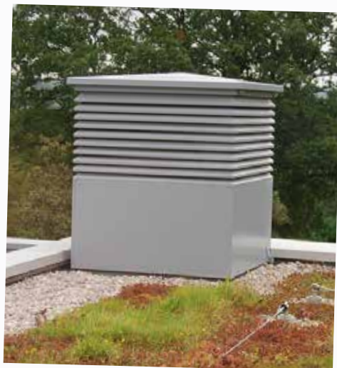
Kitchen Supply/Extract via Bespoke Windvent Style Terminal
