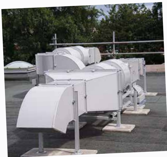
Powder Coated Rooftop Ductwork
