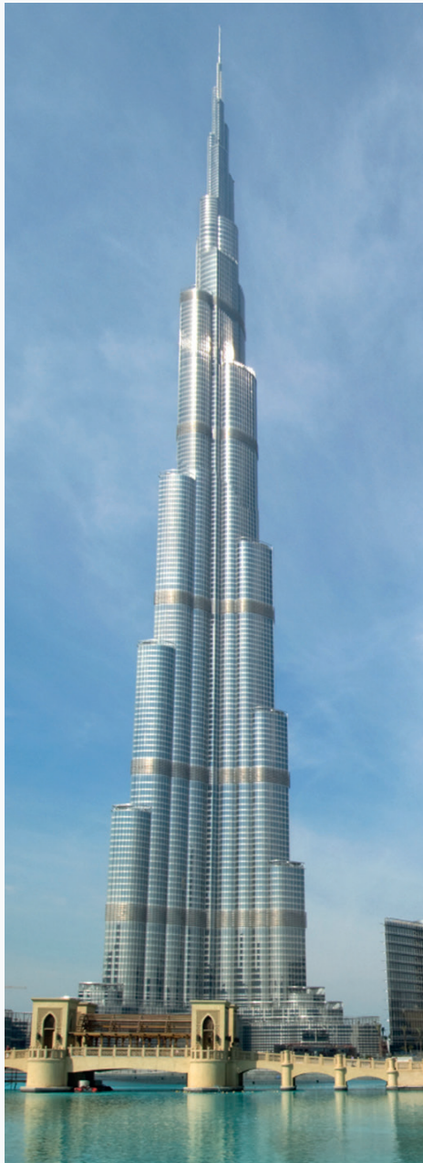
Burj Khalifa Tower over 828m high featuring 6 separate major flue systems supplied, delivered and installed by Midtherm Engineering.
