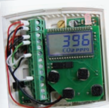
Simple internal wiring set-up
