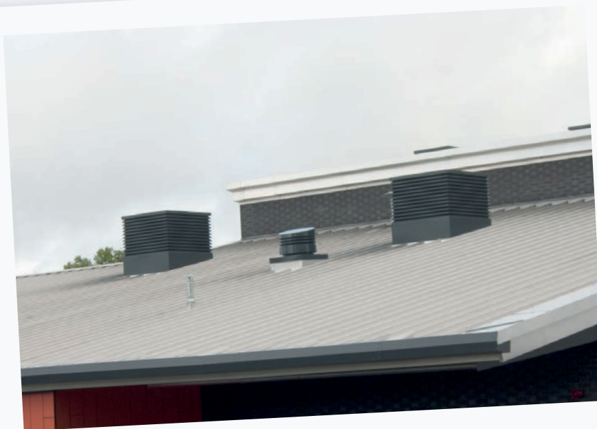
Windvent and X-Stream units in operation
