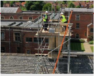
Our engineers completing a CCTV survey of the existing chimney prior to lining.
