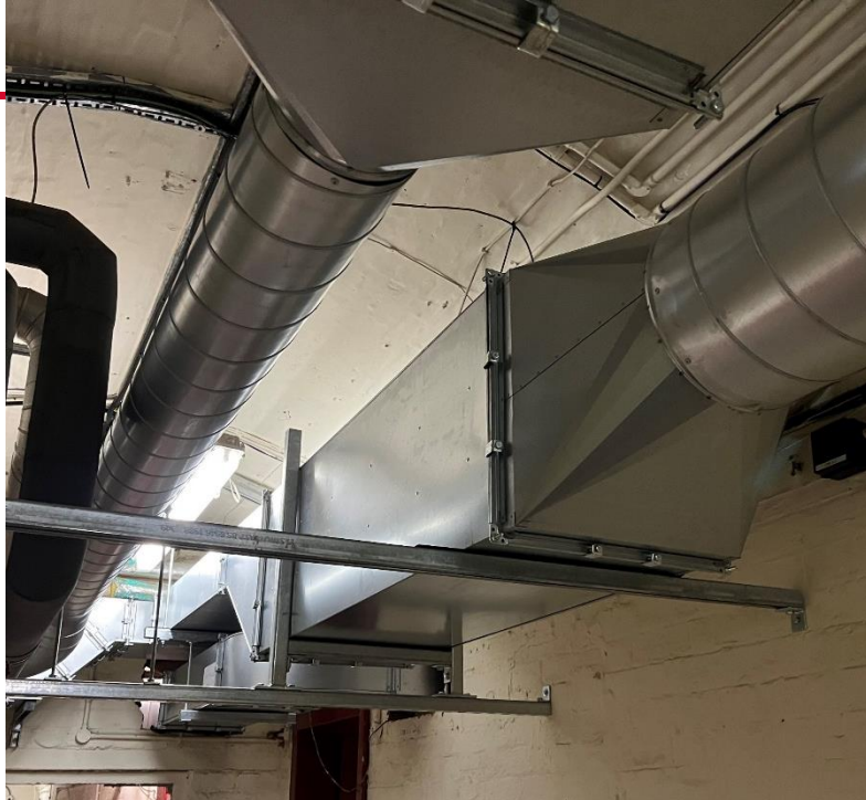
Specialist attenuation installed within our ventilation ductwork.
