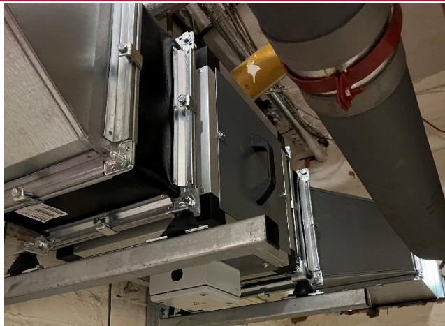
Boiler room extract ventilation fan
