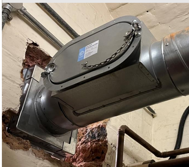
Fire damper and access hatch installed within a fire break wall.
