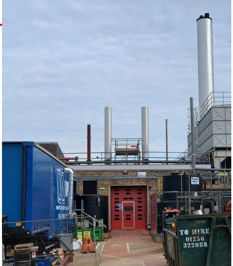
Self supporting structures in situ during installation
