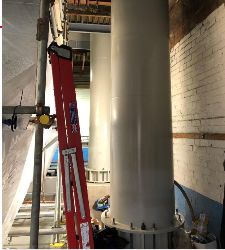
Our free standing structures positioned on their foundation blocks.
