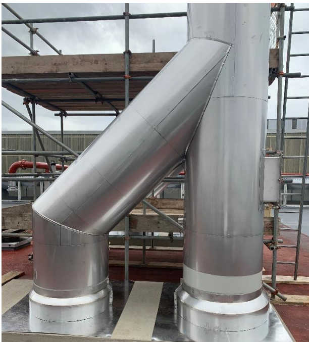
Our self supporting structures exiting the roof.
