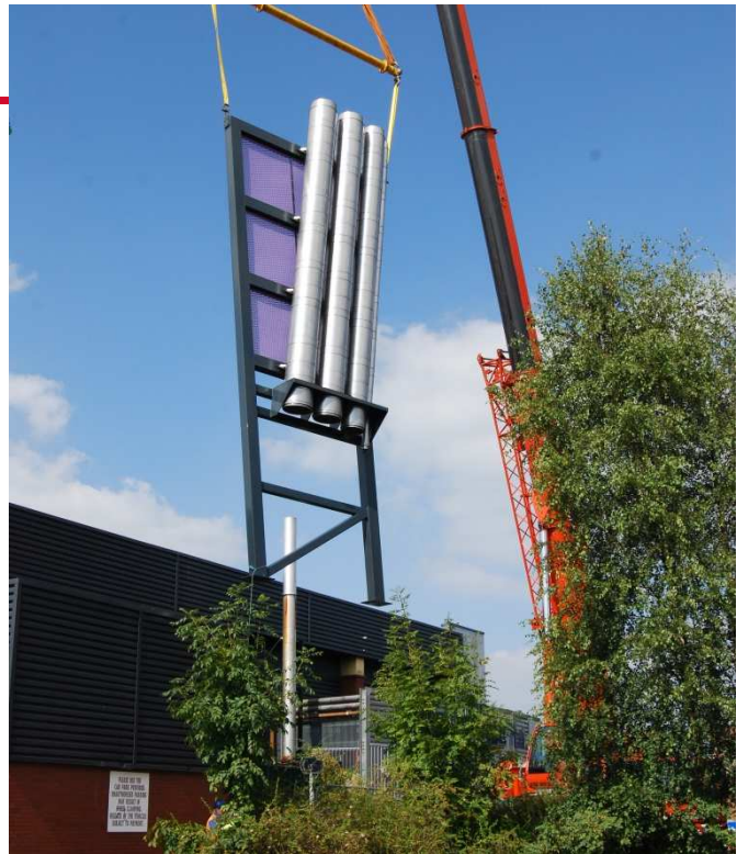
Flue and mast systems being craned into position
