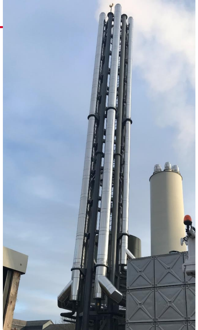
Final installation of flue systems and mast structure
